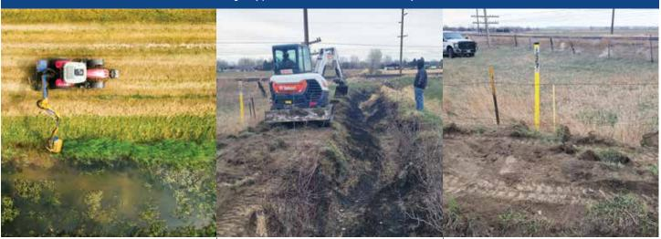
ditches require frequent maintenance due to the accumulated silt and vegetation, necessitating periodic removal to maintain the functionality.
