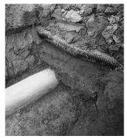
Cross at an angle as close to 90 degrees as possible and with at least 24 inches of separation. Photo Credit. Drain Tile Safety Coalition
